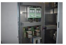
The control system was designed for a 2 cbm concrete mixing plant with the following specifications: Aggregate weigher for 5 components Lift with bucket conveyor 3000 lit. Mixer 2 cbm
